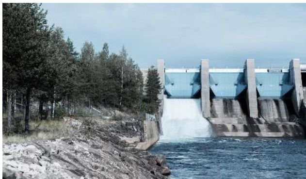
Laxede power plant, Sweden
